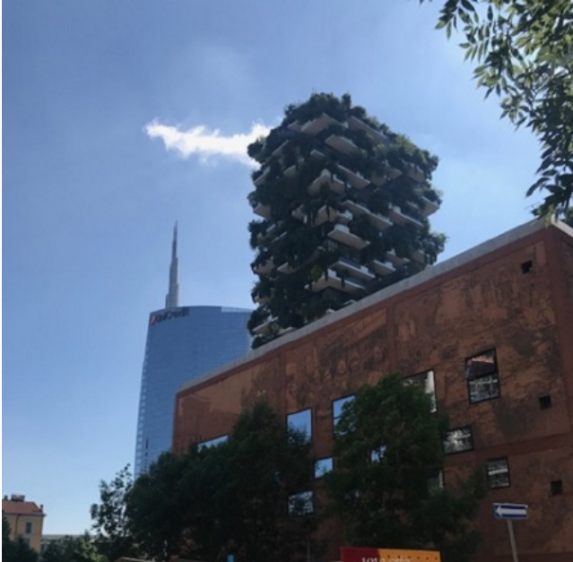
Fig. 5. The House of Memory, Bosco vertical tower and Unicredit tower (Photo by Maristella Bergaglio)
