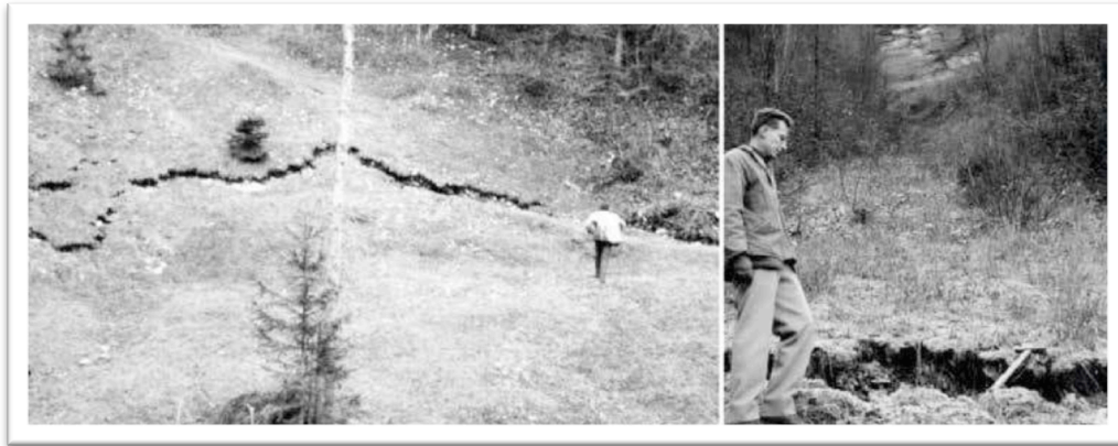
Figure 2. Fissures that appeared on Monte Toc on November 9, 1960. 16
